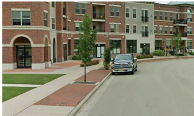
Option 1: Decorative terrace distinguishes the sidewalk from the furniture, tree and utility zone. Use of brick/pavers with a concrete base provides for authentic historic character that mitigates settling issues.
